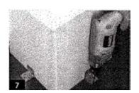
7. Obtain corner brackets from a hardware supplier. With the shaft in place, mark and pre-drill the shaft, floor and soffit to receive screws to install the corner brackets. Install screws to secure the corner brackets to the top of the shaft and the soffit and to the bottom of the shaft and the floor. NOTE: Self-tapping masonry fasteners should be used in concrete floors.
